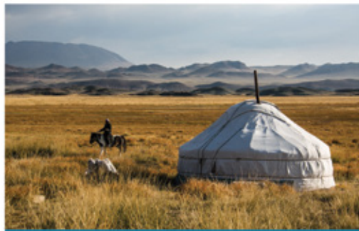
Mongolian yurts are made of skins stretched over wooden poles and can be taken apart and moved easily.
